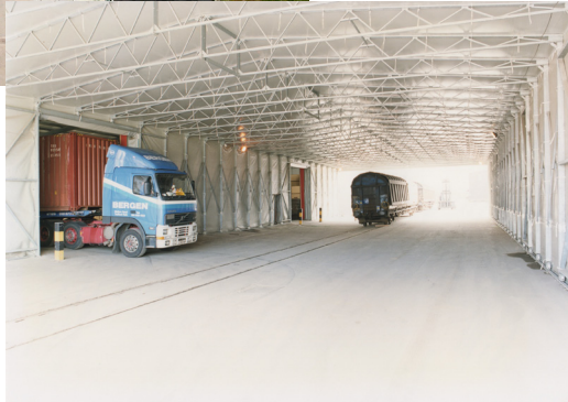
POTTER GROUP Width 15m x length 30m x internal height 5m
