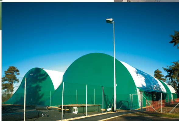
GREENACRE SPORT CENTRE 4 no. 18m wide x 36.5m long x 9m high tennis domes
