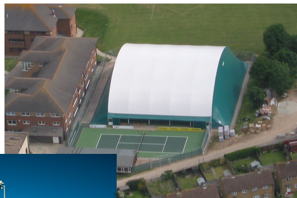
APPETI TENNIS Width 37.5m x length 37.5m x internal height 11m
