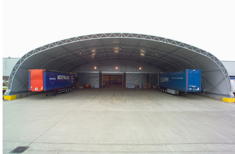
HOWDENS JOINERY Width 32m x length 22m x internal height 9m
