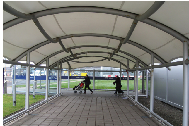
WALKWAY Width 5.8m x 3m high
