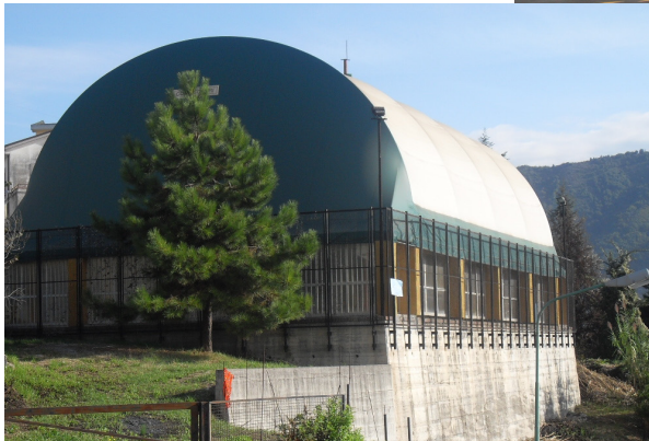
GLULAM SALT STORE Width 18m x length 25m x internal height 9m
