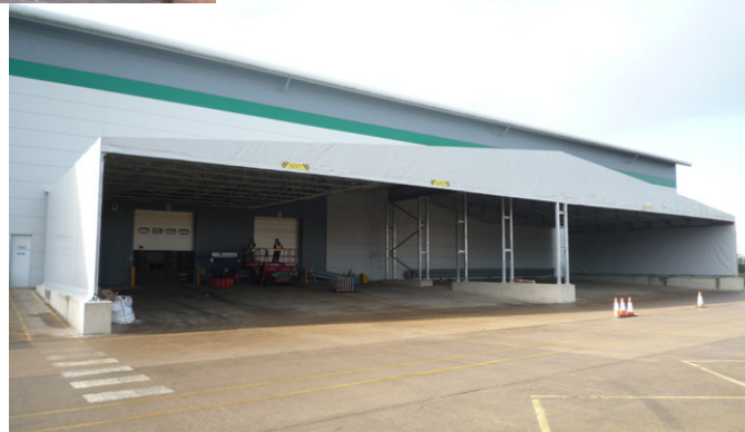
TRAVIS PERKINS Width 48m x length 18m x internal height 5.5m
